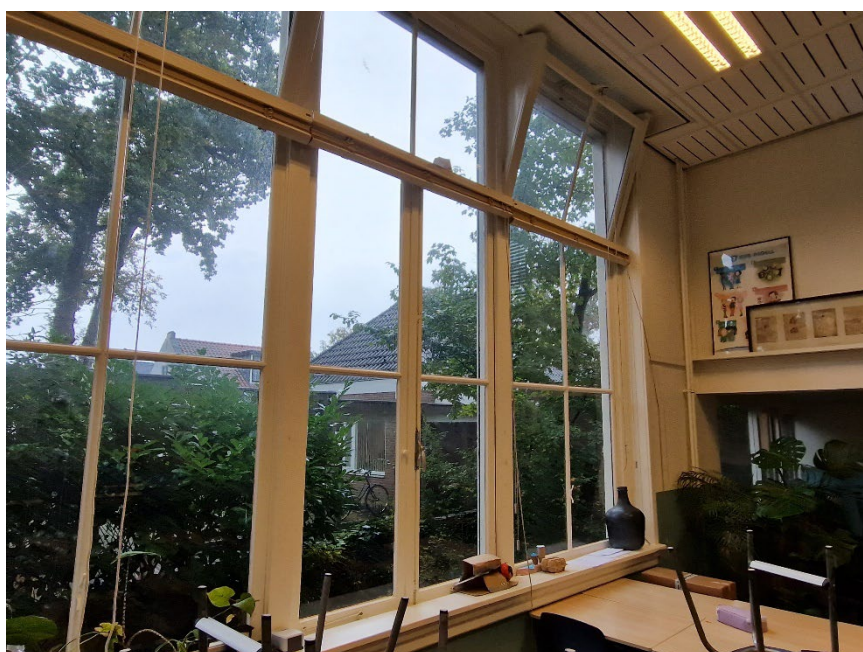
Figure 1-2 – Ventilation system before intervention
