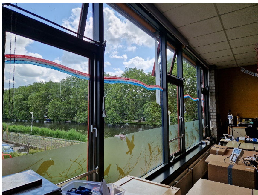
Figure 1-2 – Ventilation system before intervention
