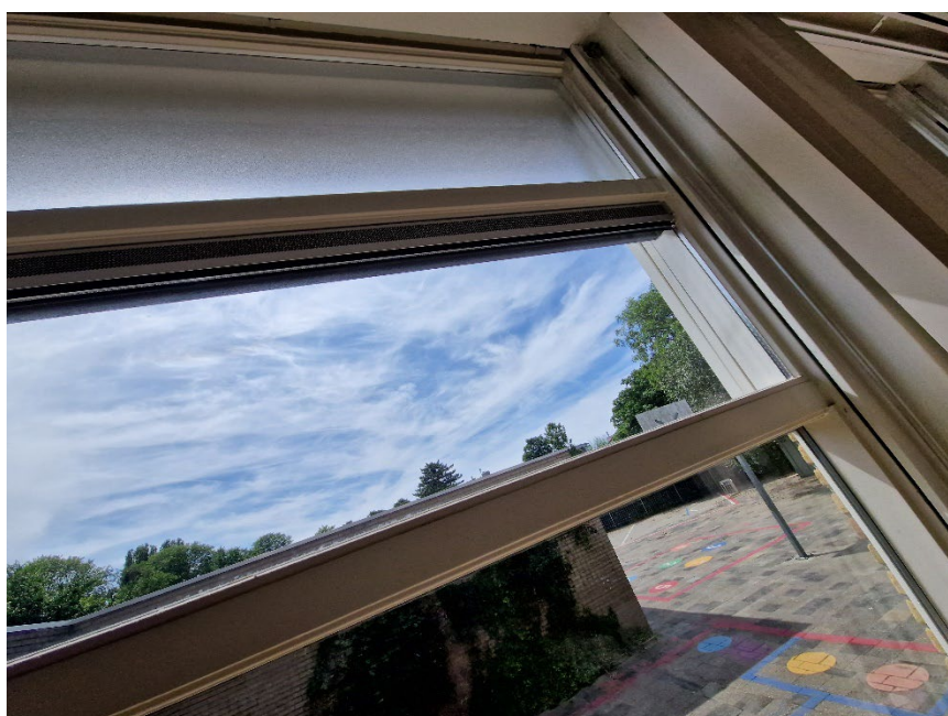
Figure 1-2 – Ventilation system before intervention
