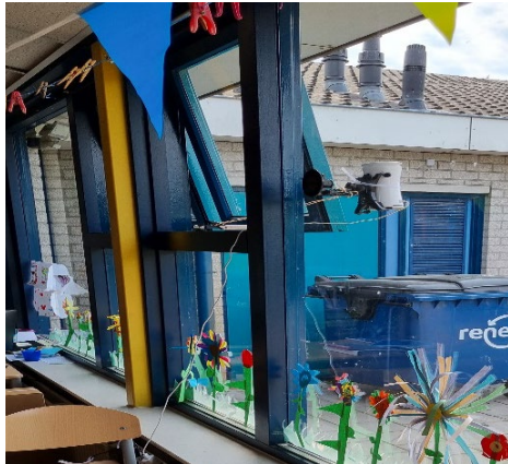
Figure 1-2 – Ventilation system before intervention
