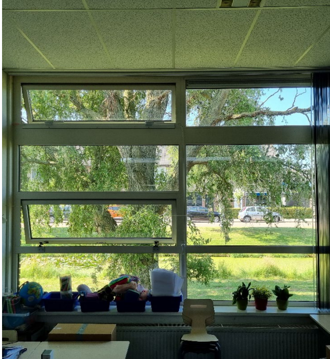
Figure 1-2 – Ventilation system before intervention
