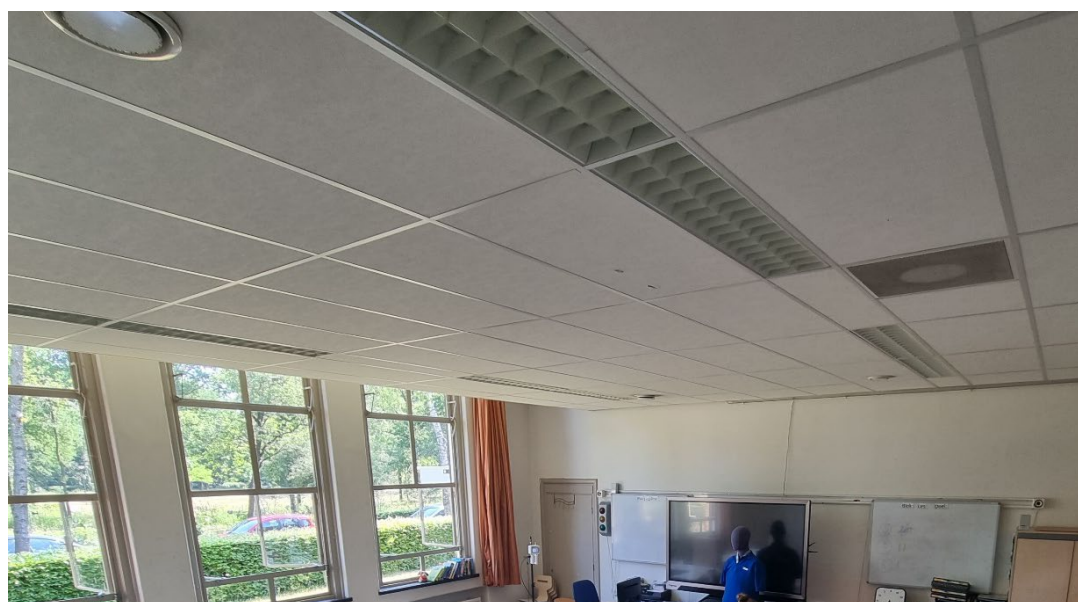
Figure 1-2 – Ventilation system before intervention
