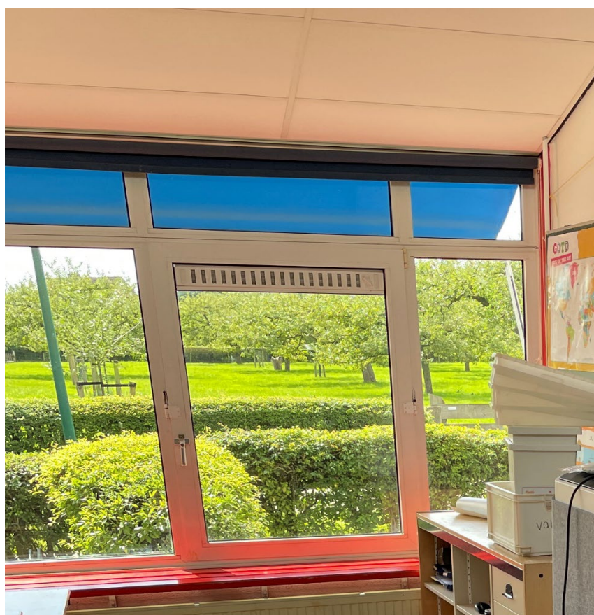
Figure 1-2 – Ventilation system before intervention
