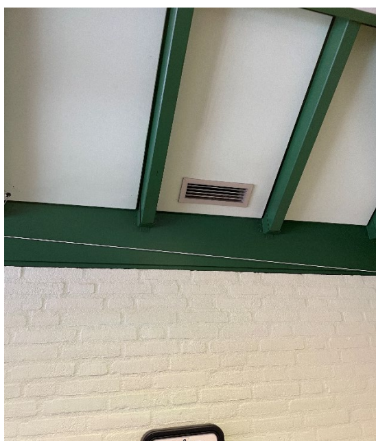
Figure 1-2 – Ventilation system before intervention
